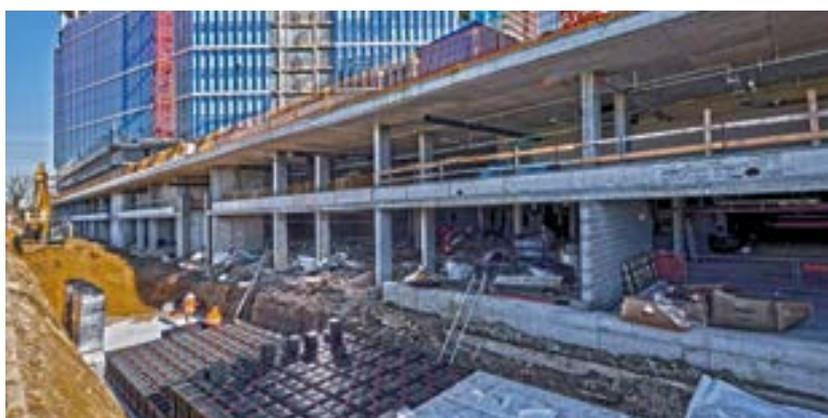
**Stormwater detention basin (1000 m<sup>3</sup>)
