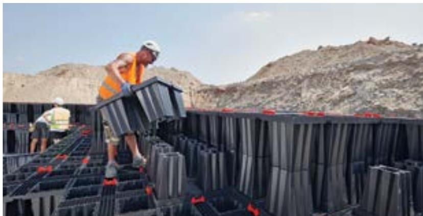
**Stormwater infiltration basin (800 m<sup>3</sup>)
