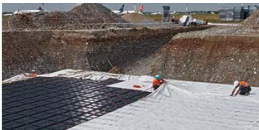
**Stormwater infiltration basin (800 m<sup>3</sup>)
