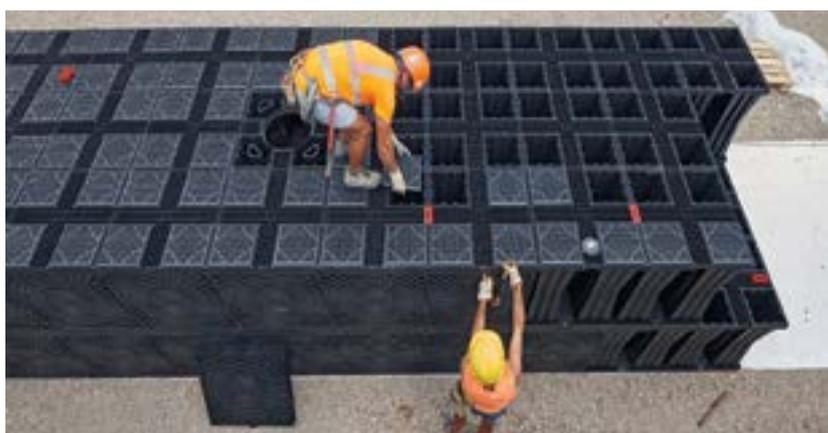
**Stormwater infiltration tank (130 m<sup>3</sup>)
