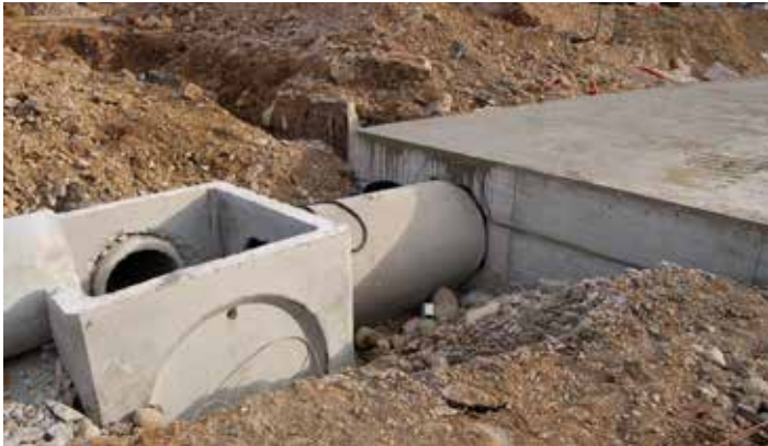
Figure 3: Particular lamination tank with lifting station.
